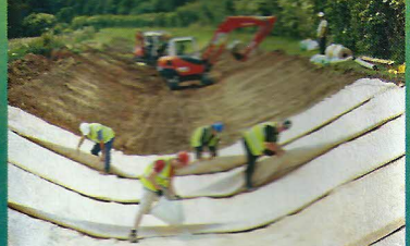
16. The liners are carefully adjusted if required, making sure they overlap.
