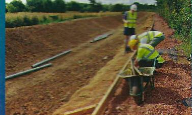
18. Coir mats, towpath boards and stone are situated before re-watering.
