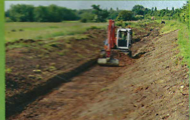
14. Re-profiling the canal bed and banks to hold water to a depth of 4ft.
