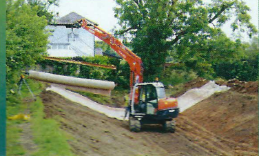
15. Bentoline SS100 Geosynthetic Clay Liner rolls are carefully applied.
